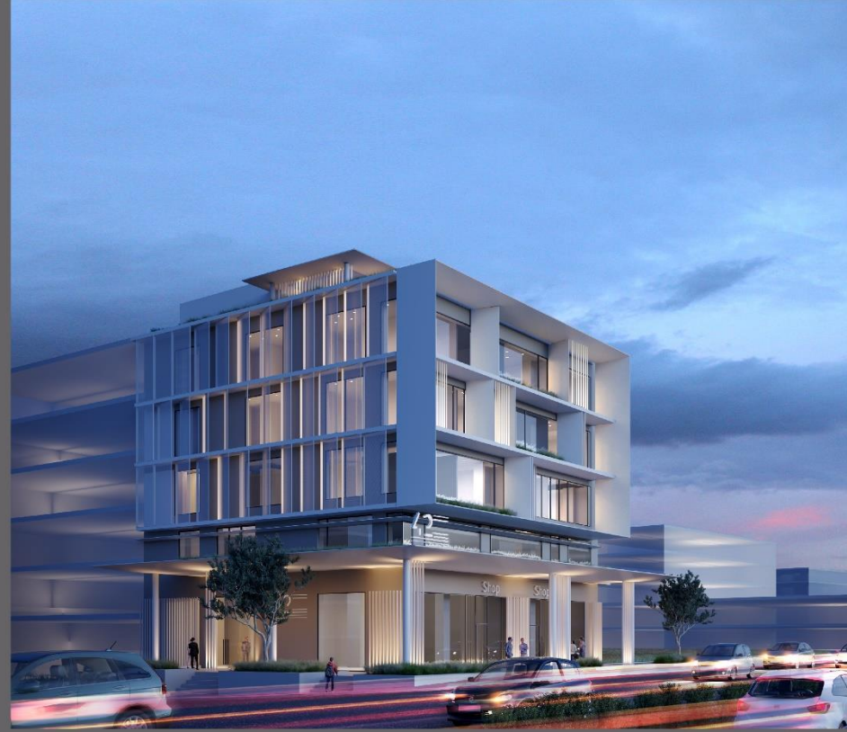
Reconstruction of office building in Kallithea, Greece
